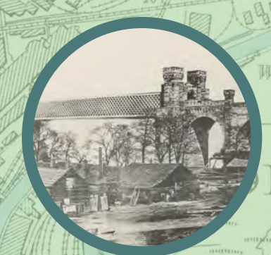
1868 Runcorn Railway Bridge
