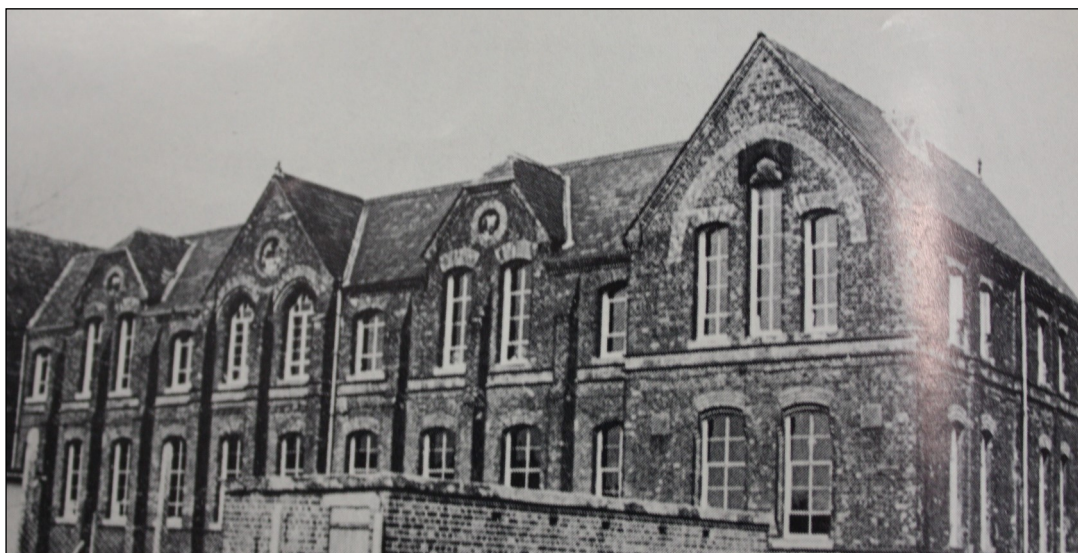
Warrington Road School pictured in Bygone Widnes G. Smith (Eaton Press, 1985) p28
